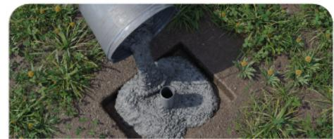
Prepare a mortar base around the tube, dimensions 40 x 30 x 10 cm.
