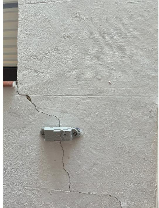
Three DELTA L+ mini sensors were installed for a six-month monitoring period.
