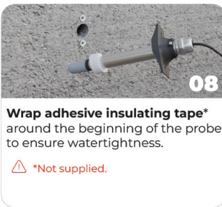
**Wrap adhesive insulating tape\*** around the beginning of the probe to ensure watertightness.
