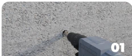
Using a drill fitted with a bit suitable for the material ( $\varnothing$  20 mm), **drill on the marked points.\***
