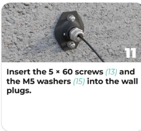
**Insert the 5 x 60 screws (73) and the M5 washers (75) into the wall plugs.**
