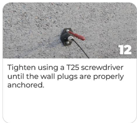
Tighten using a T25 screwdriver until the wall plugs are properly anchored.
