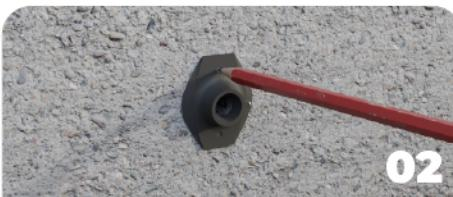
Use the Hm mounting bracket (77) to mark the drilling points.
